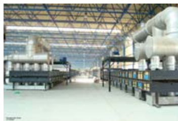
Nearing completion ... the porcelain tiles factory.
